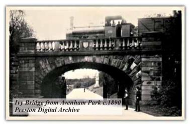
Because of the limited height it has an elliptical arch and crosses the Broad Walk between Avenham and Miller Parks on a 30 ft. skew over to the south-west, 12 ft. from the square. The parapets comprise bulbous cast iron balusters with stone copings, and alternate stone panels; there being four sets of four balusters on each parapet, with a half baluster at the end of each stone panel and parapet end.
